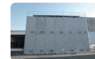
Setting up a temporary installation for dismantling
