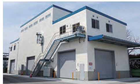
Building for pretreatment of housing/chassis/enclosure
