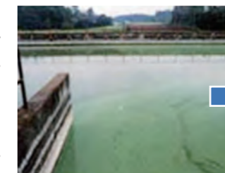
Before SHALLOW CLEAN was installed
