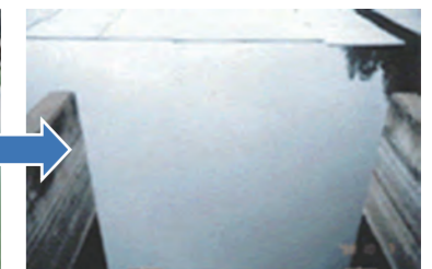
84 days after SHALLOW CLEAN was installed
