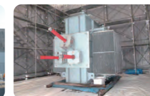
Before dismantling of waste electrical equipment
