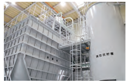
“Honestlimer”, equipment that injects a solution of calcium hydroxide (Photo provided by Kuri Water Treatment Plant, Karatsu City)
