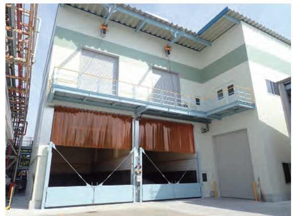
A dehydrator was added to improve wastewater treatment performance. (Photo: Expanded dehydrator building)
